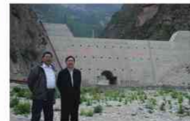
舟曲泥石流挡坝
